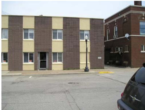
The new MOSA building, on the left, is directly behind the current MOSA building, on the right.
